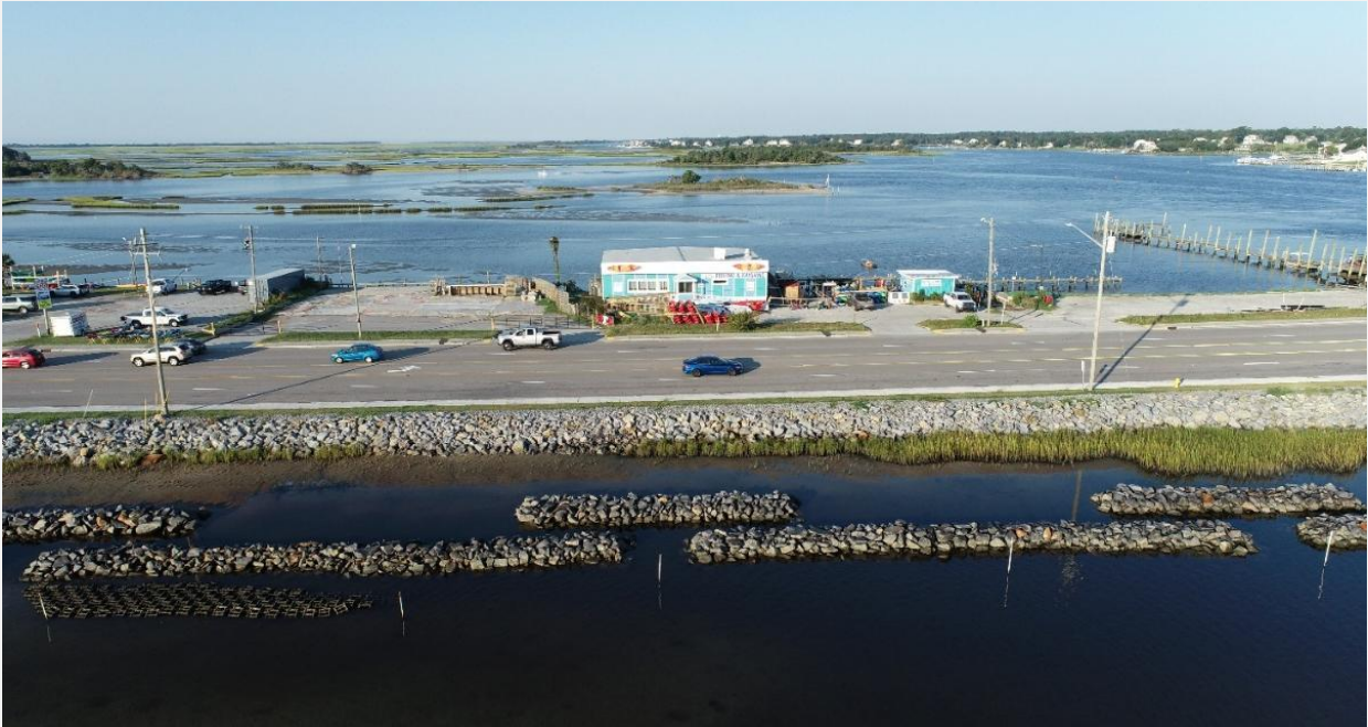
Figure 12: NC STRONG will provide new opportunities for identification of vulnerable locations that can benefit from nature-based solutions like the living shoreline NCDOT constructed along NC 24, a vital coastal route connecting Marine Corps Base Camp Lejeune.
