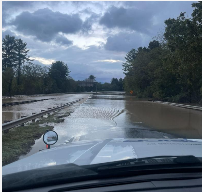
Figure 7: FIMAN alerted NCDOT to the potential overtopping of I-40 outside of Asheville nearly 48 hours in advance, allowing for planned closure of the critical route and mitigating risk to unsuspecting travelers.
